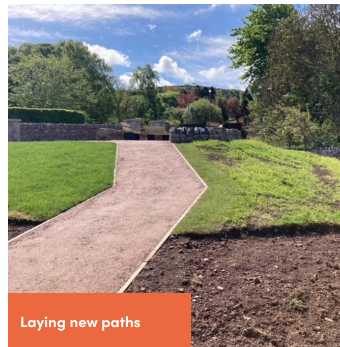
Groundworks for new paths
